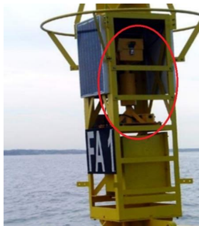
Figure 8 Example of an audible signal (Foghorn)
